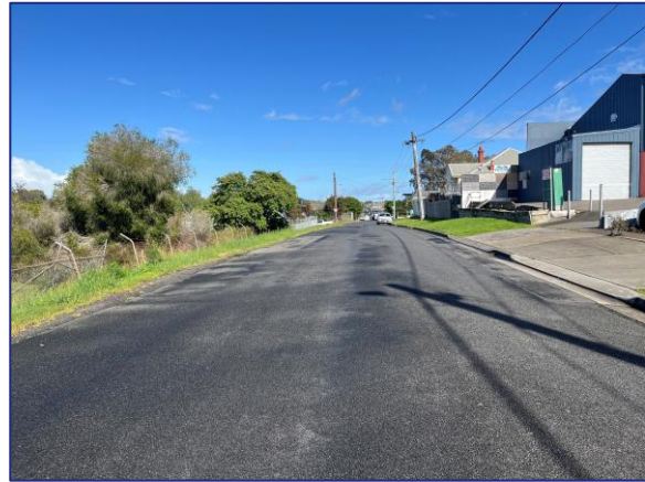
Figure 6: Little Fyans Street - view west
