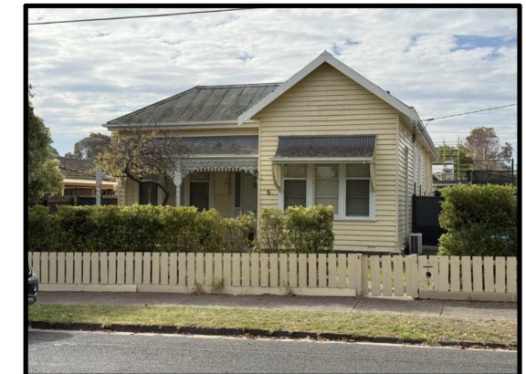
EXISTING STREETSCAPE ADJOINING DWELLING 5 TALBOT STREET
