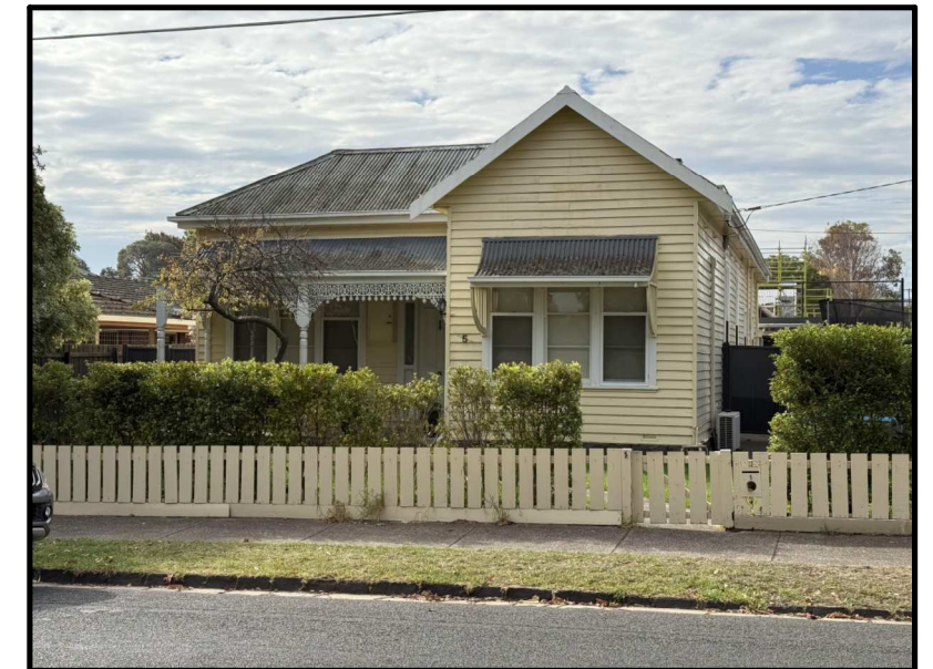
EXISTING STREETScape ADJOINING DWELLING 5 TALBOT STREET
