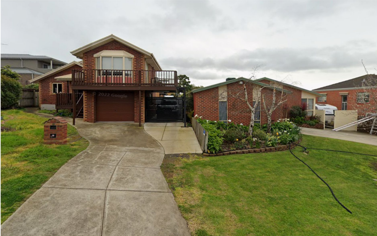
Street view image of 12 Gotemba Road.
