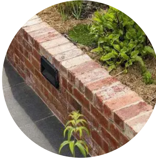
Raised brick walls to Ewing Blyth drive to provide a sense of enclosure
