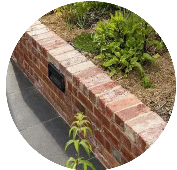
Raised brick garden beds to outdoor areas
