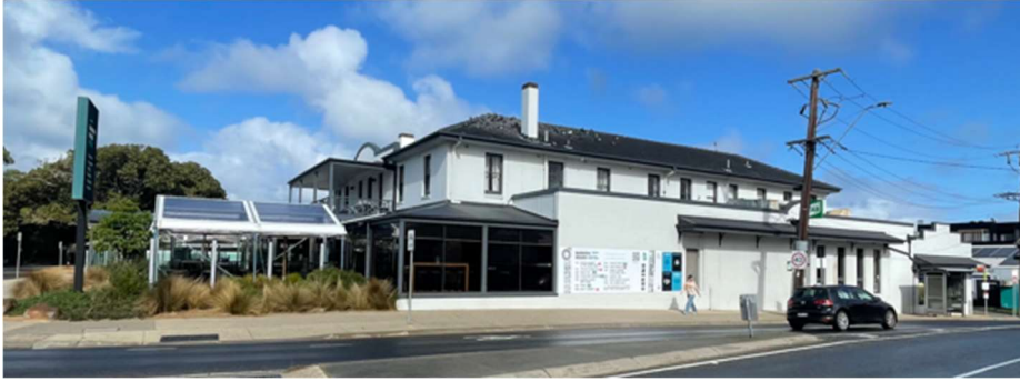
Fig 14: The existing windows and doors on the upper level of the hotel facing Bridge Road date from 1934 and are being retained. The rooms extending out to the street boundary are being demolished and the original alignment of the 1934 wall reestablished at ground floor level. (H Lardner 22/04/2025)
