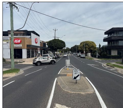
Photograph 2 – View of Bridge Road looking west
