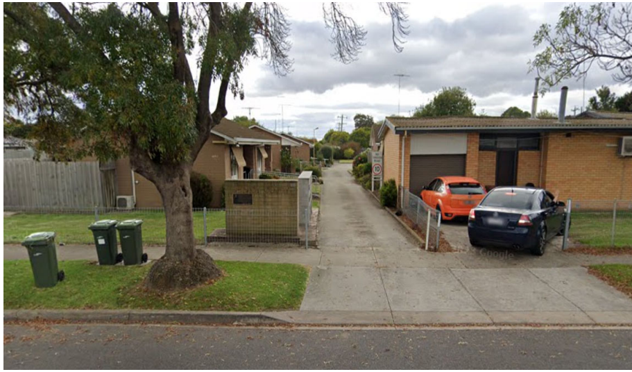
110 - 112 Sparks Rd (image Year 2023) SINGLE STOREY BRICK DWELLING CONCRETE TILED ROOF
