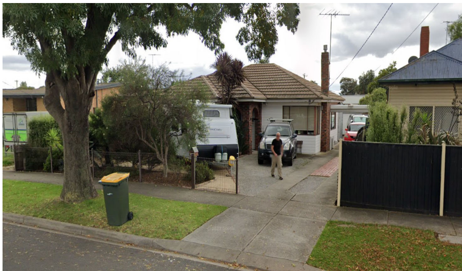
114 Sparks Rd (image Year 2023) SINGLE STOREY BRICK DWELLING CONCRETE TILED ROOF
