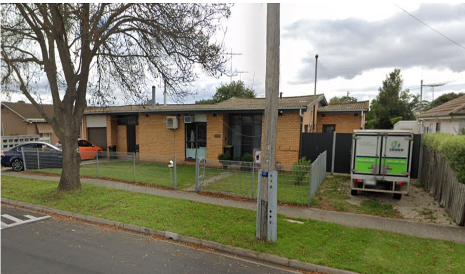
112 Sparks Rd (image Year 2023) SINGLE STOREY BRICK DWELLING CONCRETE TILED ROOF
