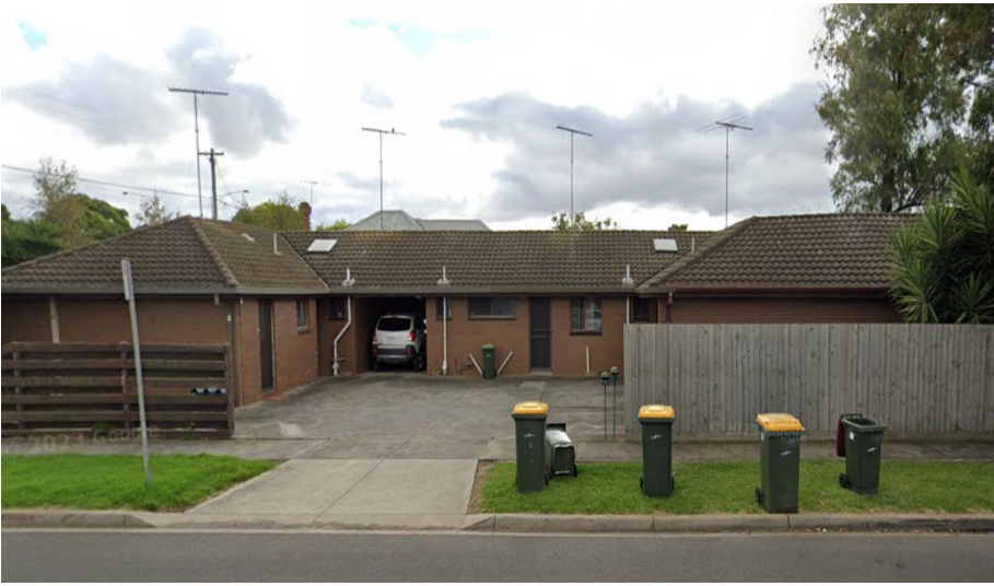
102 Sparks Rd (image Year 2023) SINGLE STOREY BRICK DWELLING CONCRETE TILED ROOF
