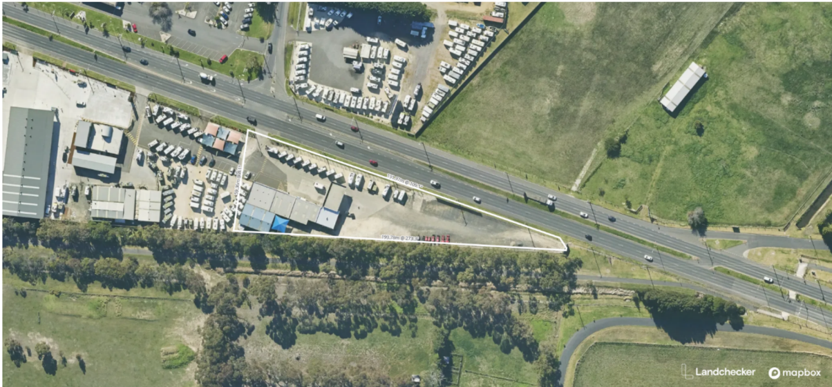
Figure 1 – Aerial Photograph of Subject Site
