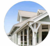
EXISTING ROOF TO REMAIN IF IN GOOD ORDER. OTHERWISE REPLACE WITH CORRUGATED SHEETING, VALLEYS AND CAPPING WITH GALVANIZED IRON. WHITE FASCIA AND GUTTER TO MATCH EXISTING
