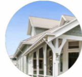
EXISTING ROOF TO REMAIN IF IN GOOD ORDER. OTHERWISE REPLACE WITH CORRUGATED SHEETING, VALLEYS AND CAPPING WITH GALVANIZED IRON. WHITE FASCIA AND GUTTER TO MATCH EXISTING
