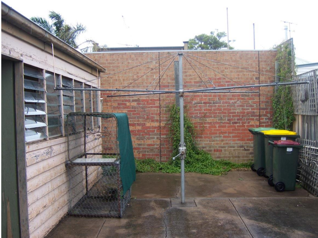
Adjacent southern property garage wall constructed to the boundary.
