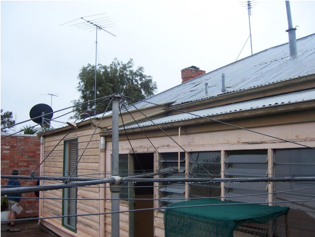
Rear section of existing building to be demolished.
