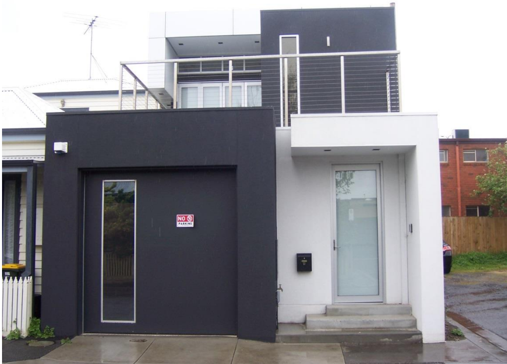
Adjacent property at 9 Cogens Pl, double storey walls constructed to the boundary.
