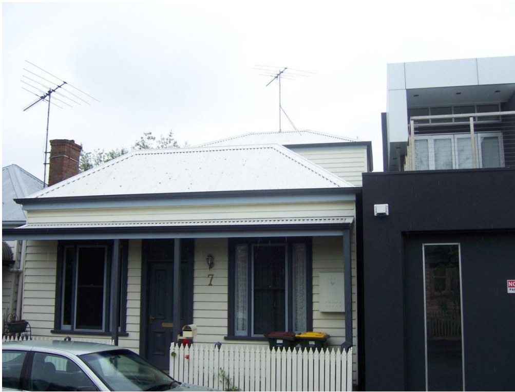
Adjacent property at 7 Cogens Pl, double storey walls constructed to the boundary.
