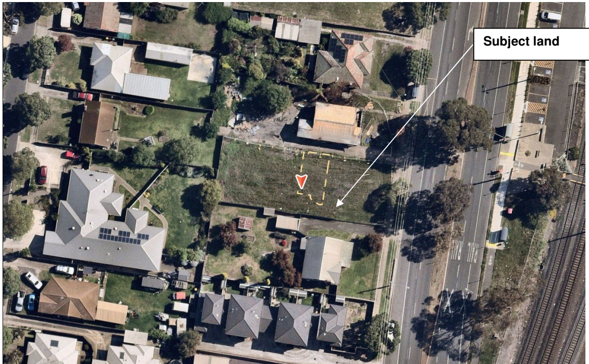
Fig 2: Aerial view of subject land.
