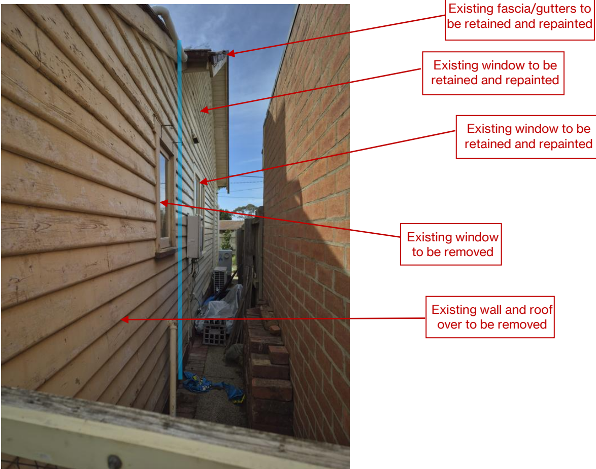
Above: View of existing south facing side (facing front of subject site). Existing laundry proposed to be removed (not part of original dwelling) and lounge and bedroom walls, window and roof over proposed to be retained. The proposed works include new paint to cladding, window trims etc and fascia/gutters.
