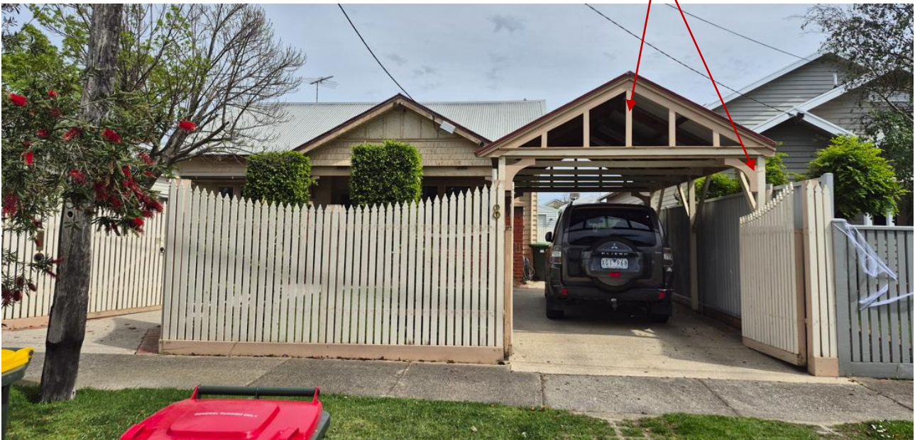
Above: View of existing carport proposed to be retained and repainted.
