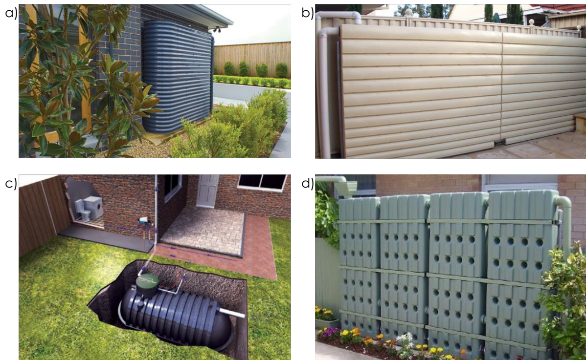
Figure 7 - Types of Rainwater Tanks a) Slimline; b) Storage walls; c) Underground; d) Modular ( www.yourhome.gov.au/water/rainwater & www.freshwater.com.au )
