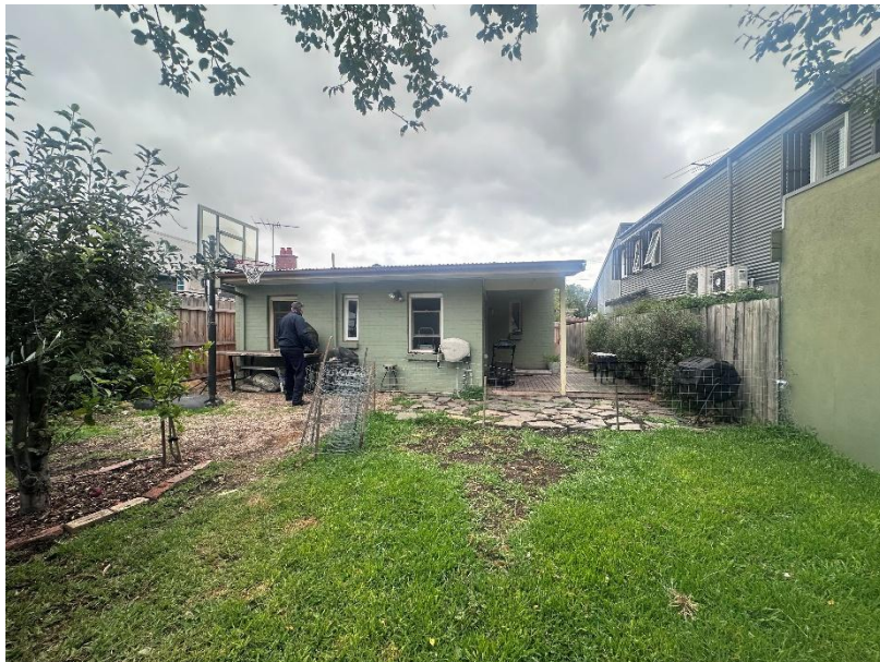
Looking north toward the flat roofed extension
