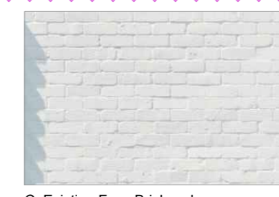
C. Existing Face Brickwork
