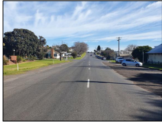
Figure 7: Fenwick Street – view west
