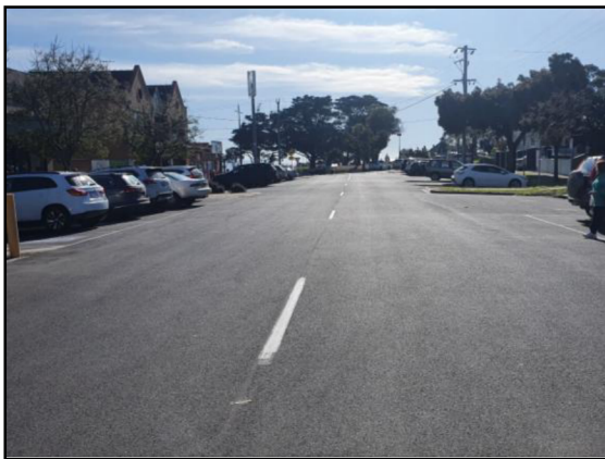
Figure 4: Brown Street - view north
