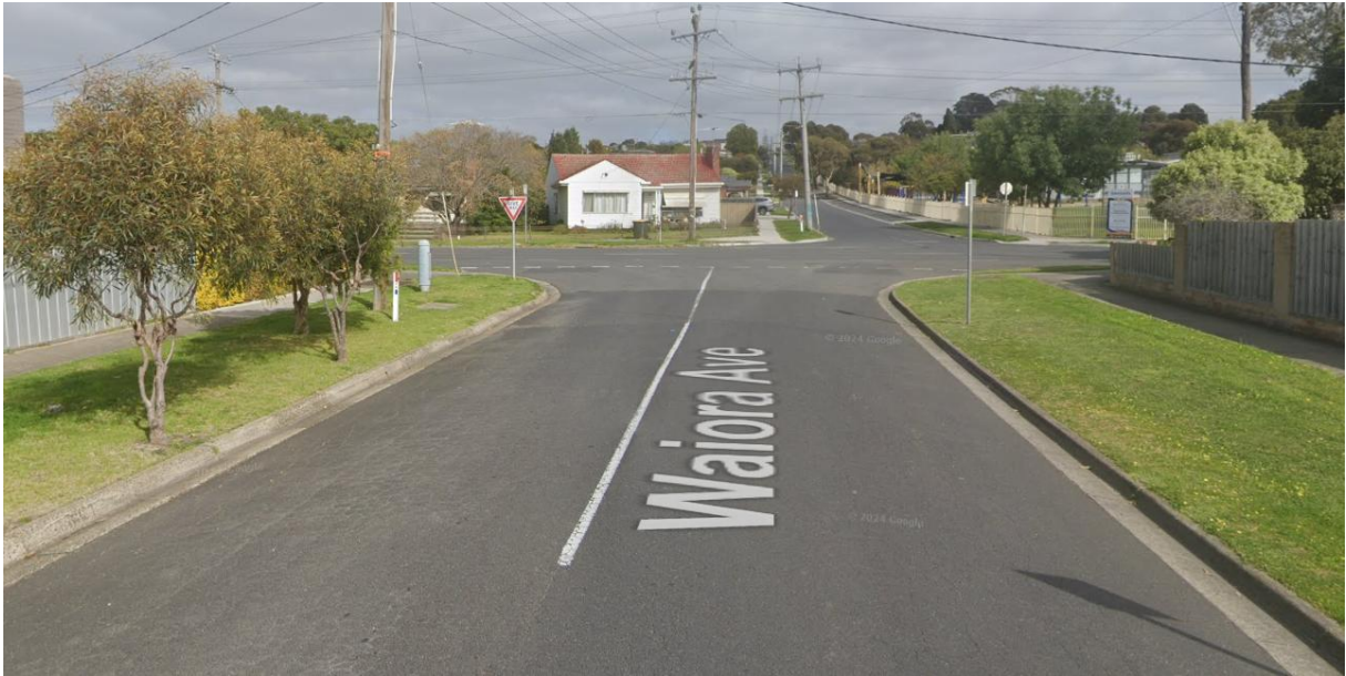
Figure 2-4: Waiora Avenue facing West
