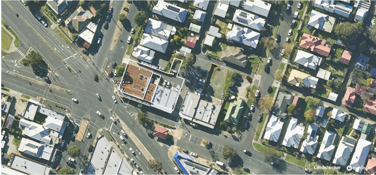
Figure 1 – Aerial Photograph of Subject Site
