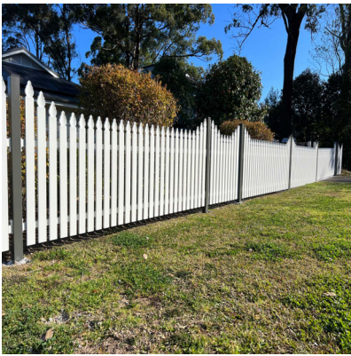
Front fence pickets and posts to be painted in Dulux Hog bristle quarter matt
