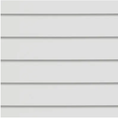
Existing weatherboard cladding to be painted in Dulux Hog bristle quarter matt
