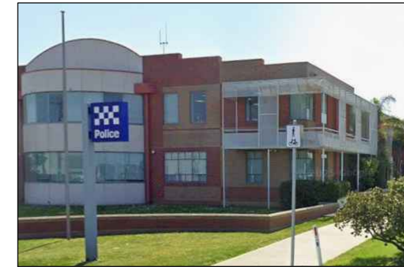
Corio Police Station
