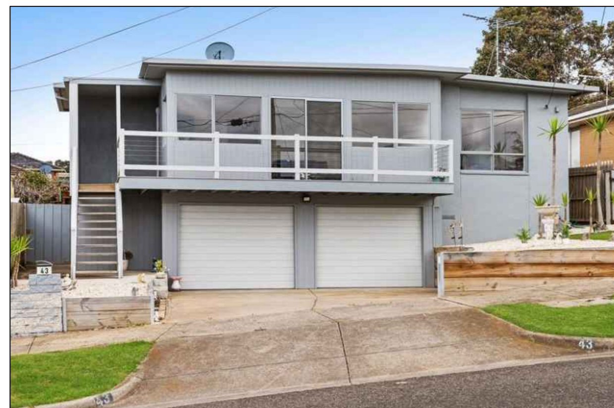
43 Kansas Ave - Across Road
