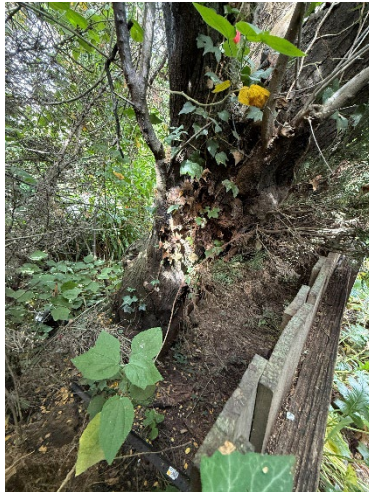
Base of Tree 18 showing advanced borer activity
