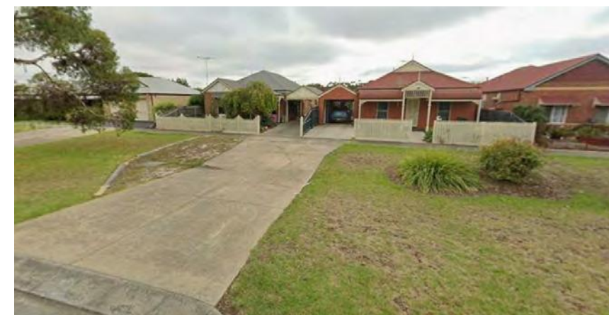
27 + 29 ARCHIMEDES AVE - SHARED DRIVEWAY ON 3-LOT SITE
