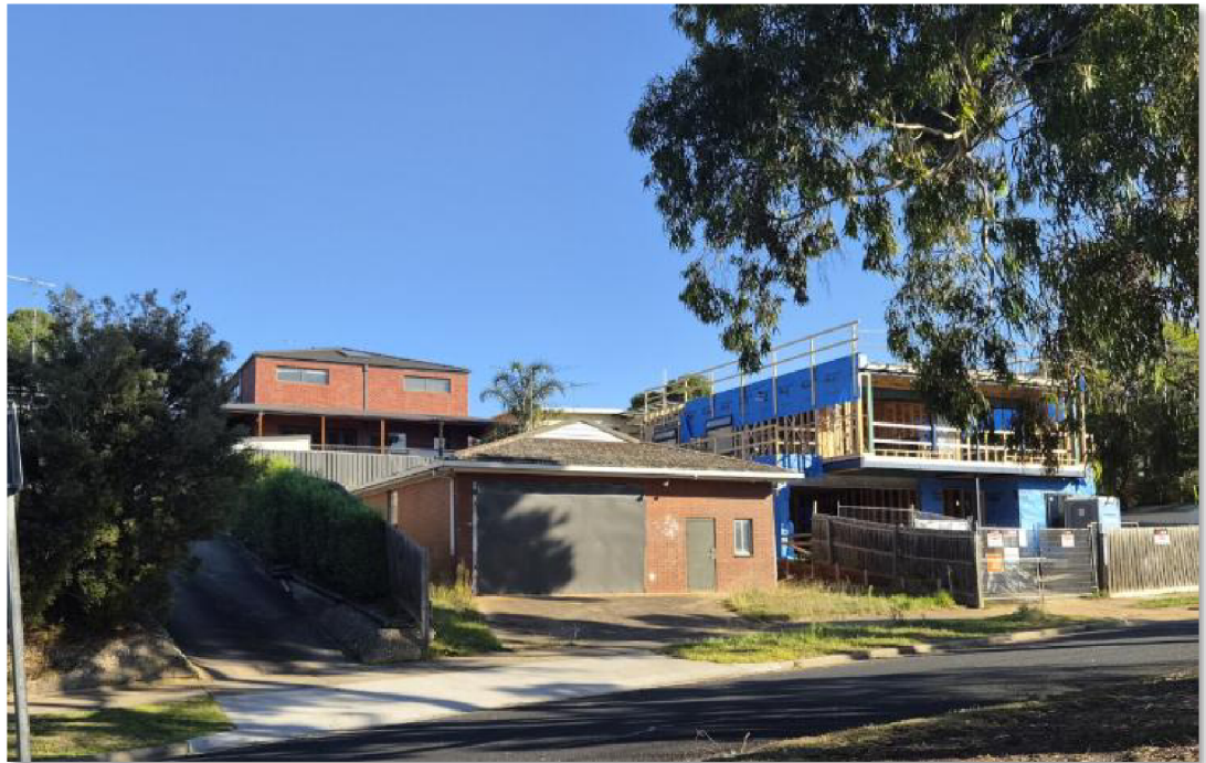
Development being undertaken at 65C Edison Avenue, Bell Post Hill
