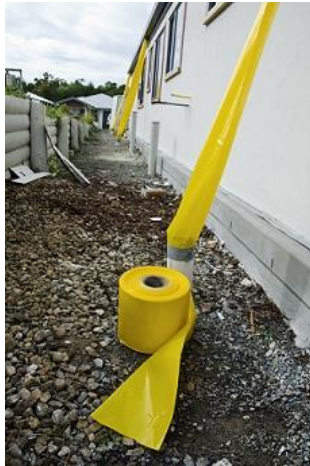
Figure 2 - Temporary Downpipes
