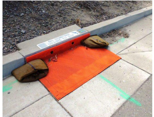
Figure 3 - Sediment Trap
