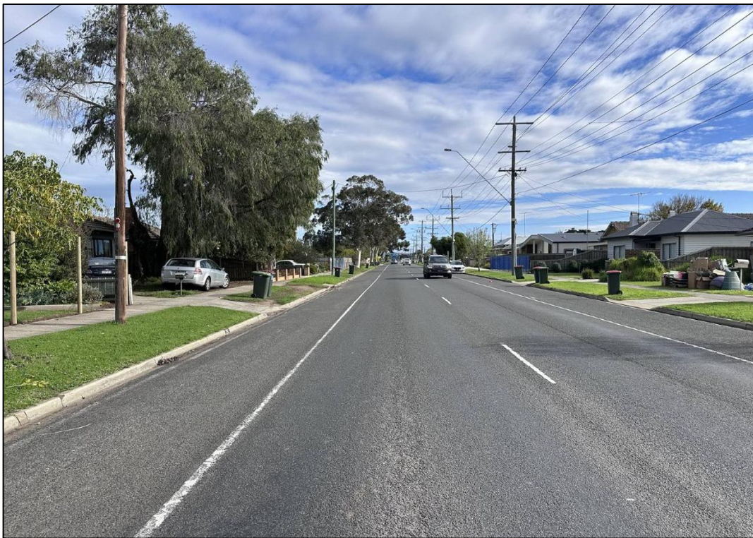
FIGURE 5: TOWNSEND ROAD, FACING WEST
