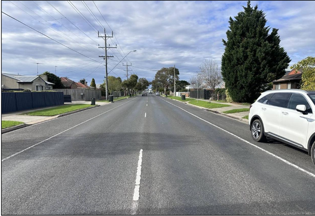
FIGURE 4: TOWNSEND ROAD, FACING EAST
