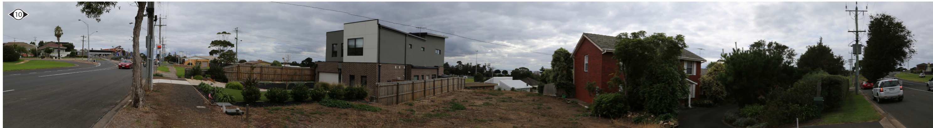
Figure 10 Panoramic view from the front of 5 Newcombe Street
