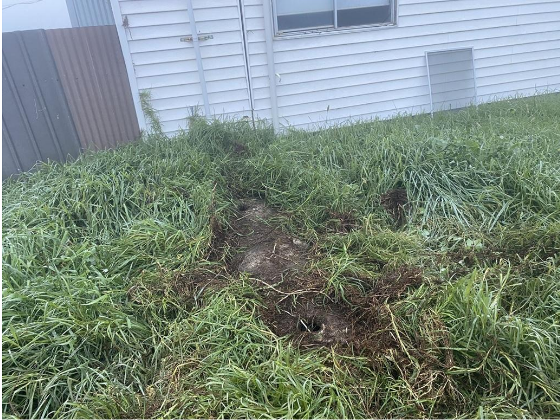
Top of primary septic tank at existing residence.
