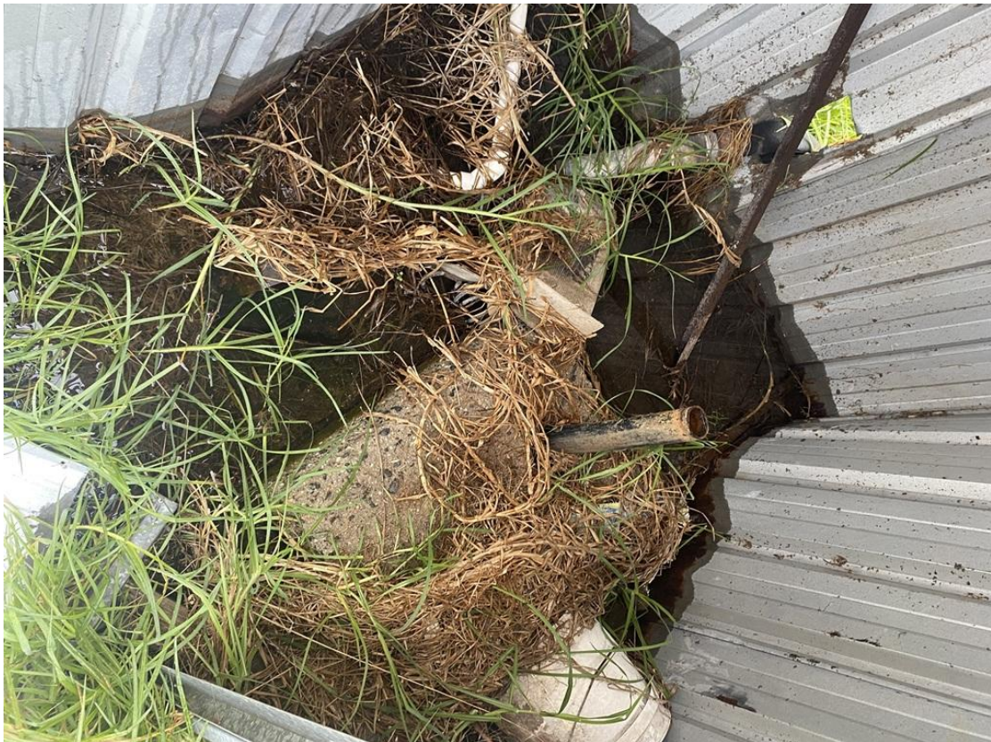
Borehead of disused waterbore.
