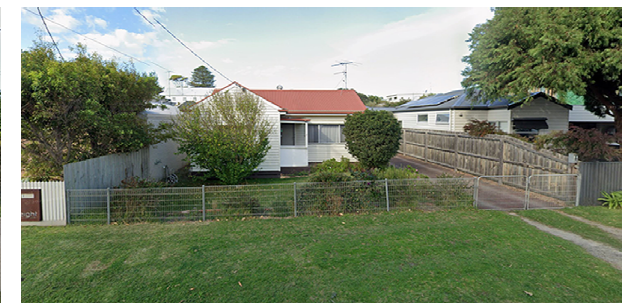
6 MARGATE STREET 1-STOREY WEATHERBOARD DWELLING
