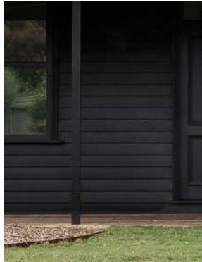
EXC3 EXISTING TIMBER WEATHERBOARDS BLACK
