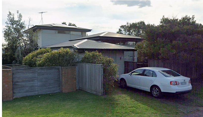
1 MARGATE STREET 2-STOREY WEATHERBOARD DWELLING
