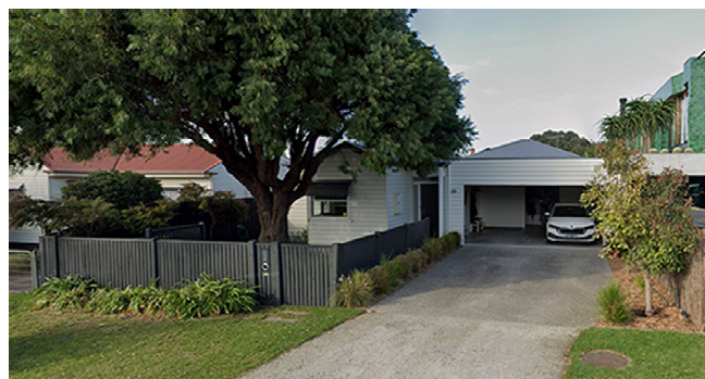
4 MARGATE STREET 1-STOREY WEATHERBOARD DWELLING
