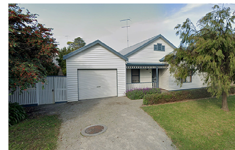
8A MARGATE STREET 1-STOREY WEATHERBOARD DWELLING
