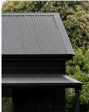
EXR1 EXISTING CORRUGATED METAL ROOFING BLACK
