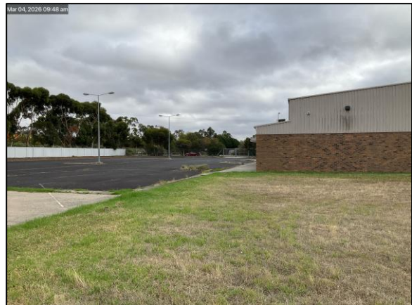
Photo 4. View looking north west from the rear of the site towards Purnell Road.
