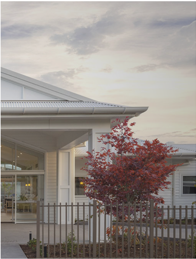
WARNERS BAY - NSW ARCARE WARNERS BAY - NSW ARCARE ARRIVAL EXPERIENCE
