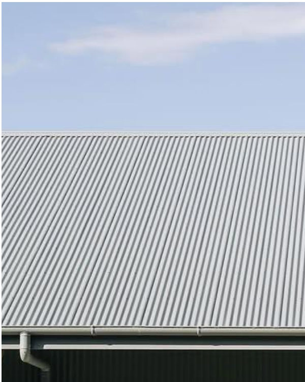
LIGHT COLOURED CORRUGATED ROOFING
