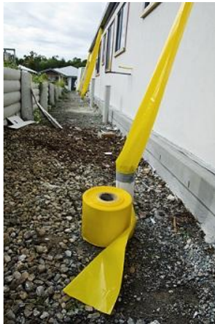
Figure 2 - Temporary Downpipes
