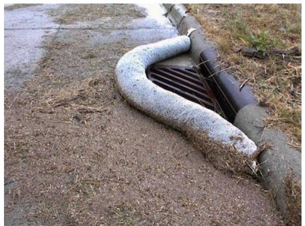
Figure 5 - Sediment Trap
