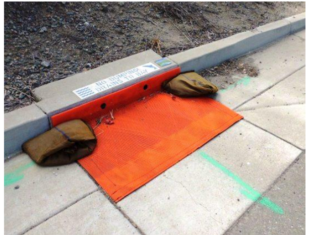
Figure 3 - Sediment Trap
