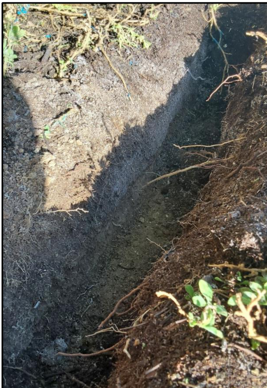
Figure 6. Poor soil structure and no viable roots from tree 1 were identified.
