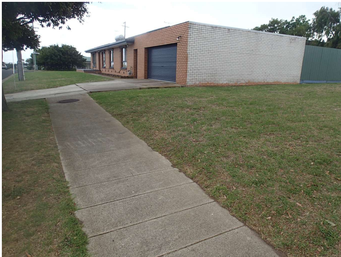
North Neighbour - On site 39 Henderson Street at the front boundary looking north.
