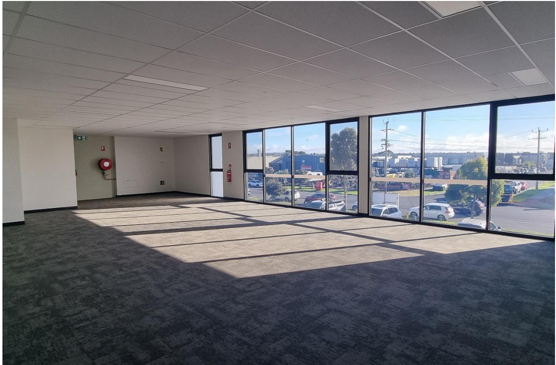
Image 7: View of mezzanine first floor level (looking north-west).
