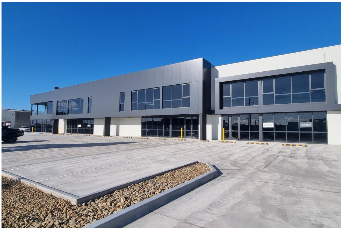
Image 2: View of Site frontage, access and car parking areas (looking south-east).
