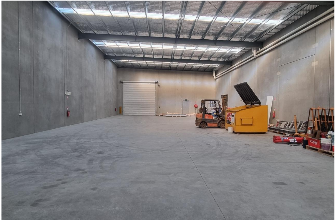
Image 5: View of ground floor and rear/southern entrance (looking south).
