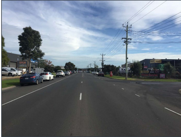
Figure 3: Marshalltown Road (View West)
