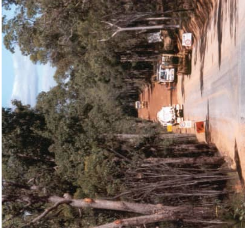
Road construction with Phytophthora Dieback infected soil or gravel can lead to the introduction of the disease to adjacent bushland.
