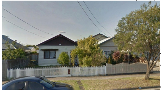
Existing timber Weatherboard house to be extended
