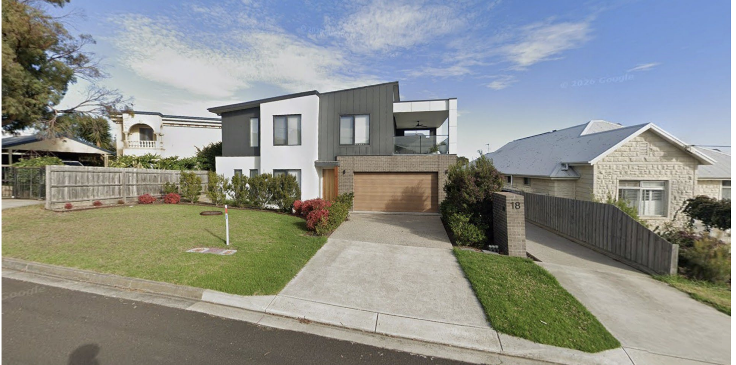
Figure 5 – Surrounding unit development at 18 Reaby Street Portarlinton
