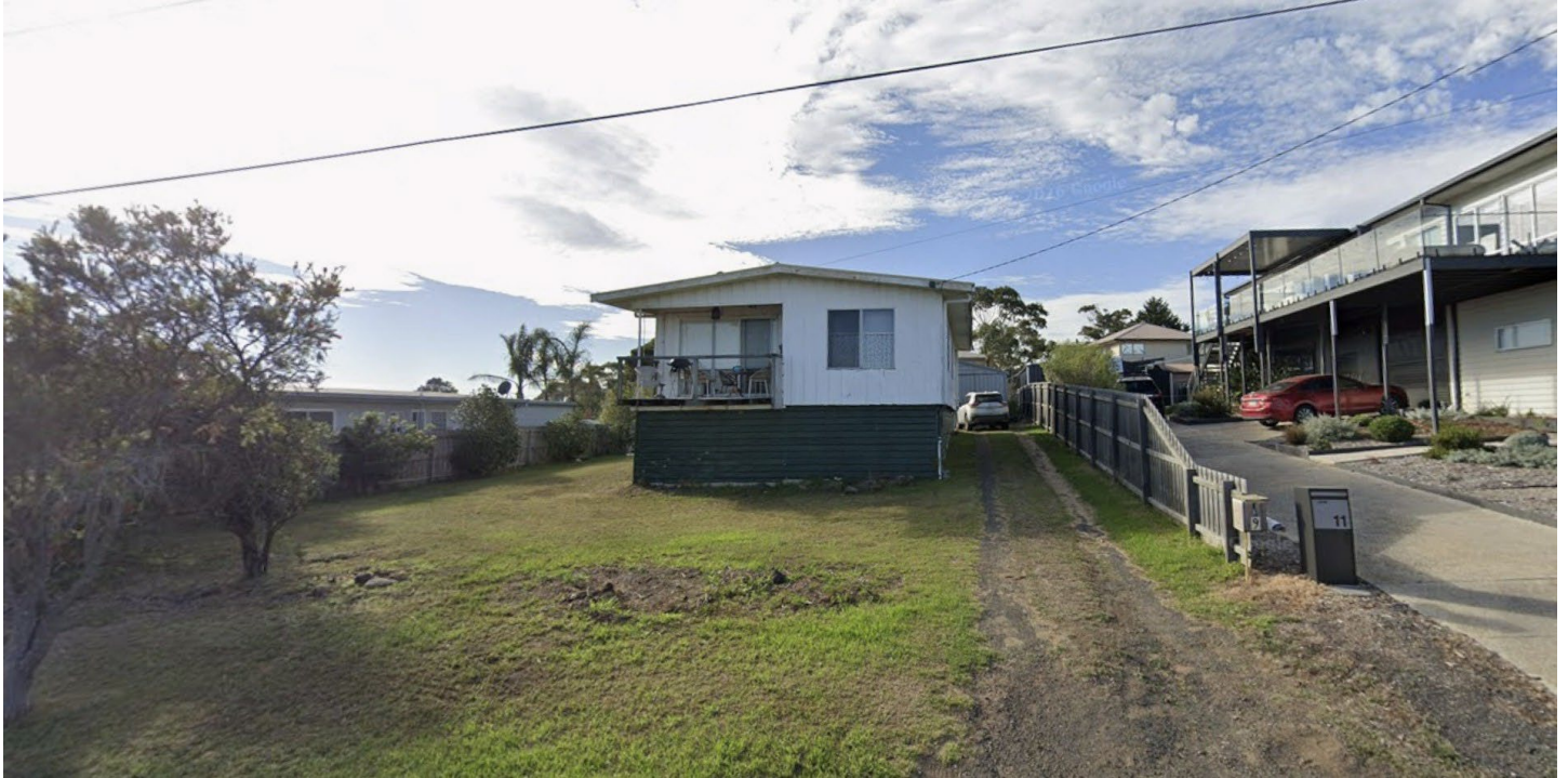
Figure 3 – Streetview of 9 Reaby Street Portarlington
