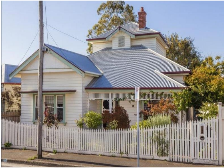
Figure 10 — 112 Skene Street, Newtown. Neighbour two doors east (subject site to left). Double storey weatherboard with hip roof. Second storey visible from Skene street.
