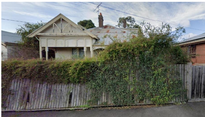
Figure 9 — 7 Cumberland St, Newtown. Neighbour immediately east (subject site to right). Two storey weatherboard with hip roof. Second storey towards the rear.
