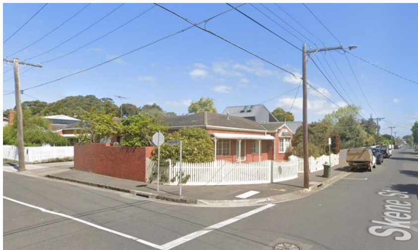
Figure 11 — 107 Skene Street, Newtown. Neighbour diagonally opposite. Non contributory brick house with hip tiled roof.
