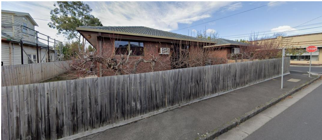
Figure 5 — Subject site, Existing Cumberland Street Frontage with high fence
