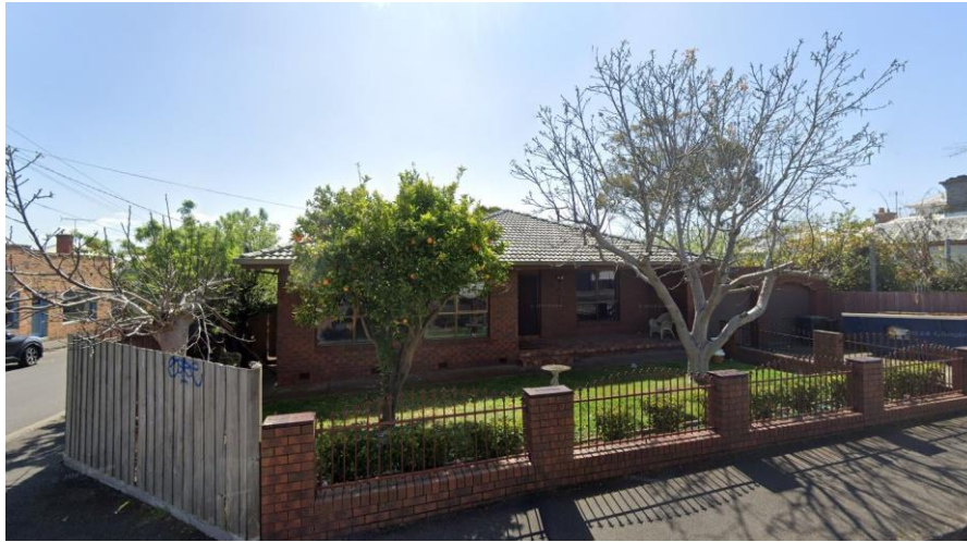
Figure 4 — Subject site, Existing Skene Street Frontage
