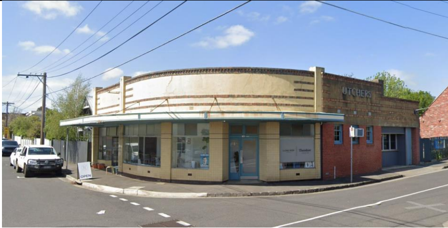
Figure 7 — 1/105 Skene Street, Newtown. South neighbour on south side of Skene st. (Subject site immediately opposite) Skene st. Atypical Post War Commercial Building at Zero setback
