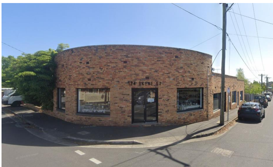
Figure 6 — 124 Skene Street, Newtown. West neighbour on west side of Skene st. Subject site to right over Cumberland. Atypical Post War Commercial Building at Zero setback
