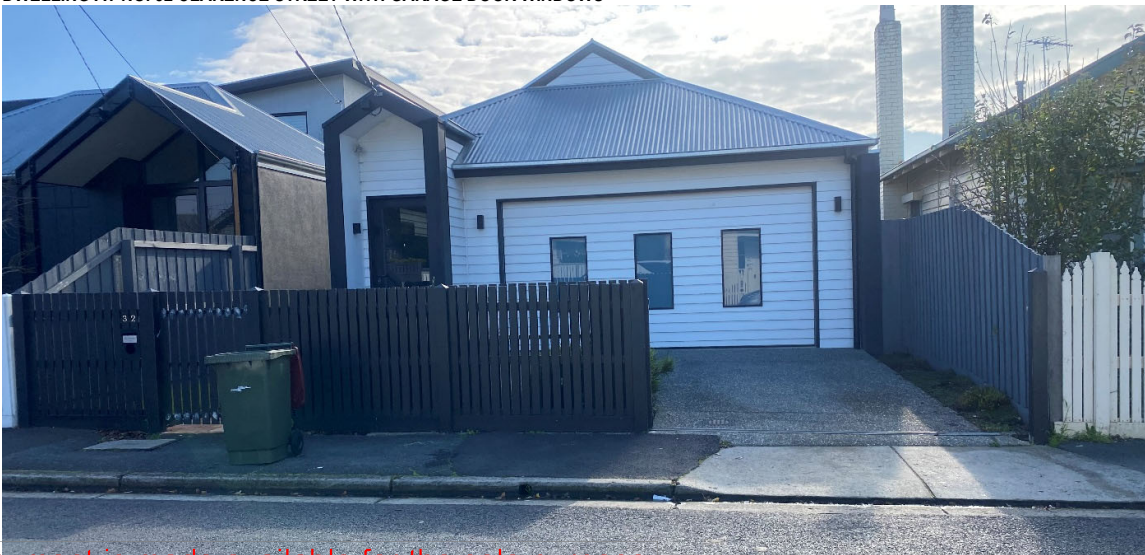
DWELLING AT NO. 32 CLARENCE STREET WITH GARAGE DOOR WINDOWS
