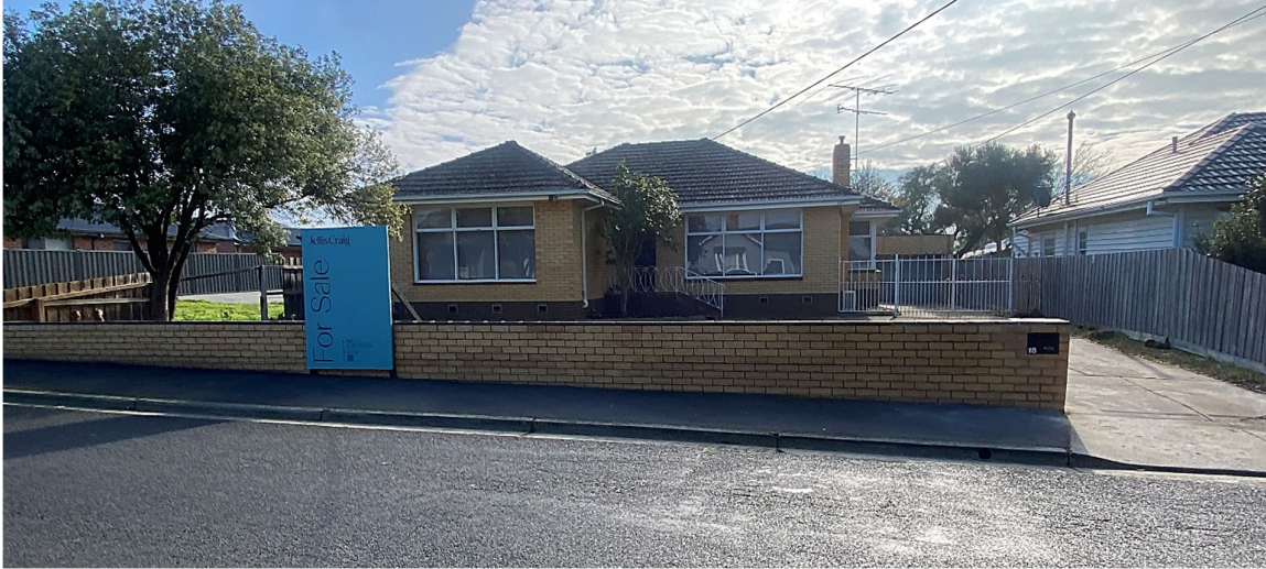
PHOTO – ADJOINING DWELLING TO THE EAST AT 18 CLARENCE STREET
