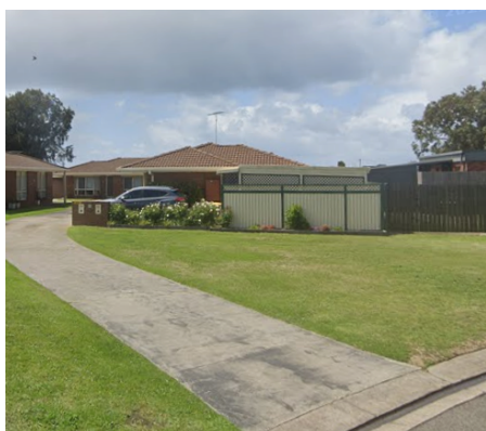
1/15 Seaforth Drive – supplied photograph
