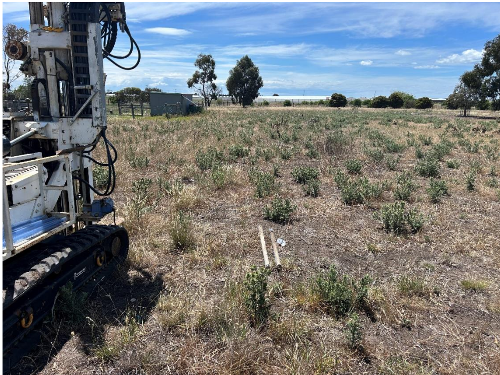
4. Proposed Effluent Field – facing east
