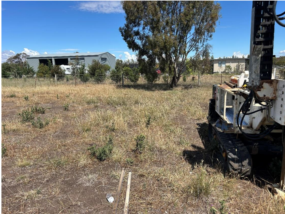
1. Proposed Effluent Field – facing west
