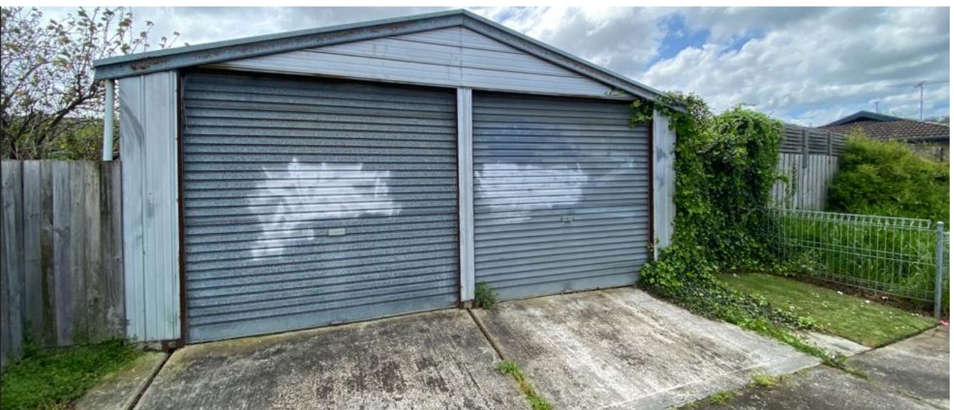
Photograph 3: Existing galvanised iron garage
