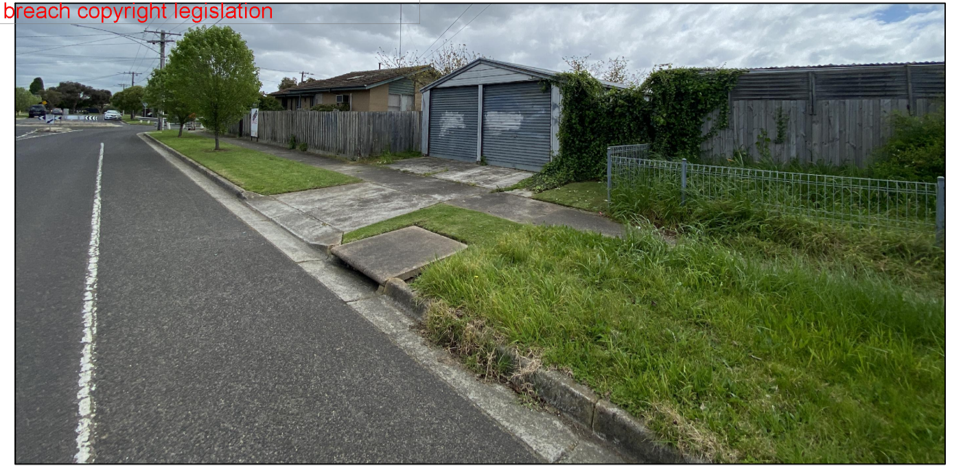
5 The existing vehicle crossings are conveniently located and are suitable for retention as part of any development application.
