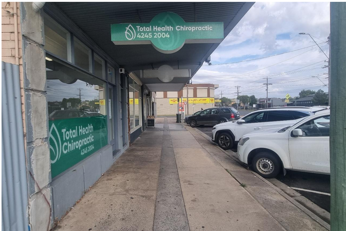
Image 2: View of adjoining frontage and footpath (looking north-west).
