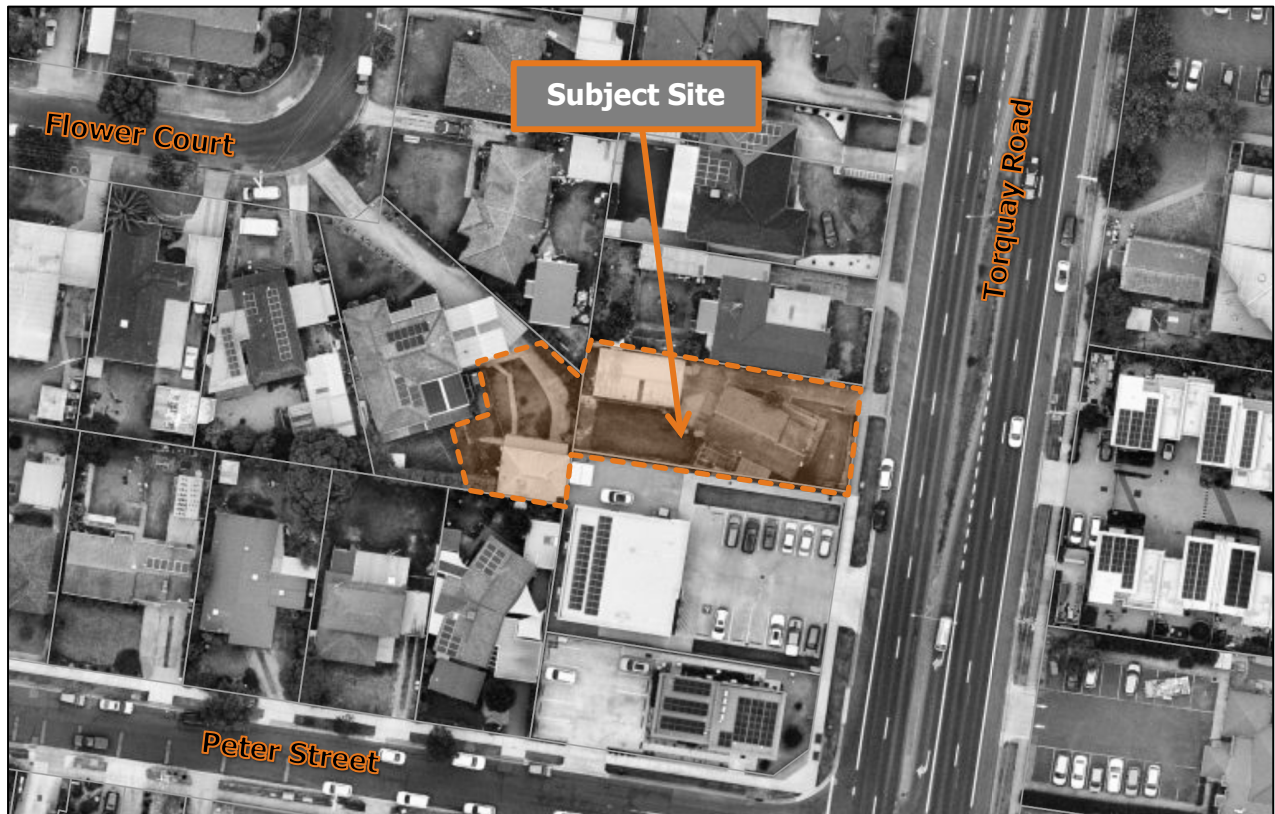
Figure 1: Aerial Photograph (source: www.nearmap.com )
