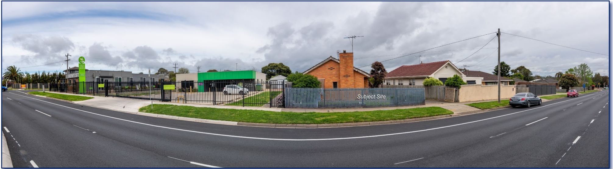
FIGURE 1 - WEST SIDE OF TORQUAY ROAD
