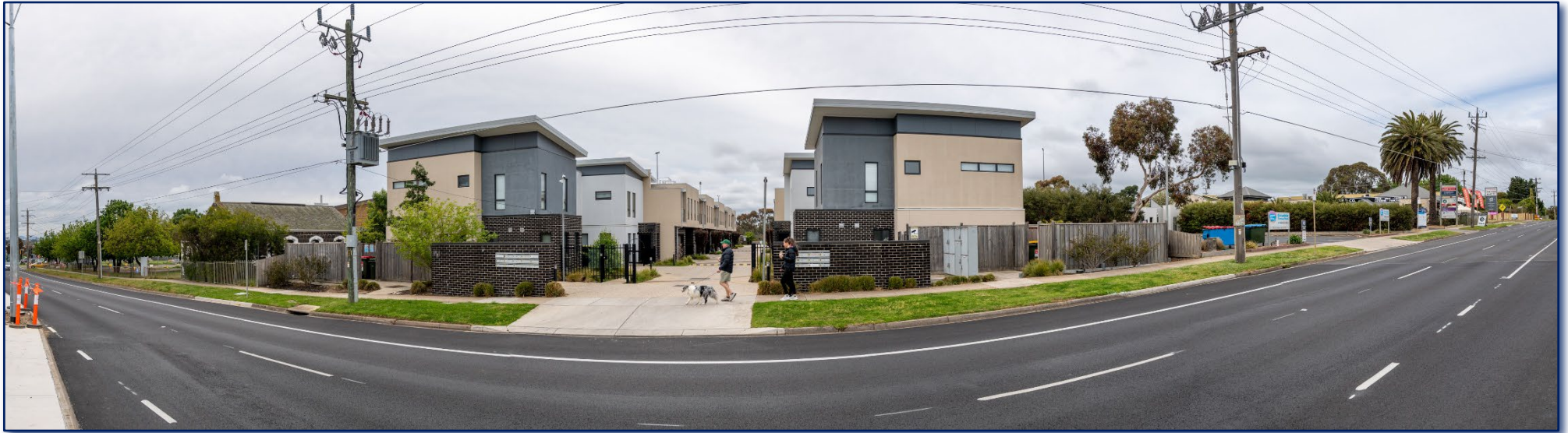
FIGURE 3 - NORTH SIDE OF TORQUAY ROAD
