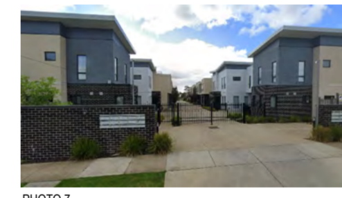
PHOTO 7 No 284 DOUBLE STOREY BRICK AND RENDERED BUILDING FLAT / GI ROOF TOWN HOUSES
