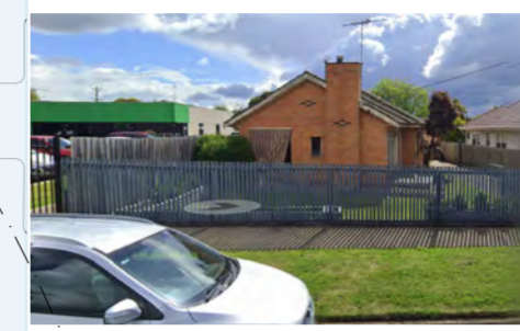
PHOTO 3 No 279 TORQUAY ROAD SUBJECT SITE EXISTING SINGLE BRICK DWELLING TO BE DEMOLISHED
