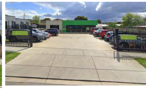
PHOTO 2 No 281 TORQUAY ROAD EXISTING SINGLE RENDERED CONCRETE COMMERCIAL BUILDING - GROVE FAMILY HEALTH
