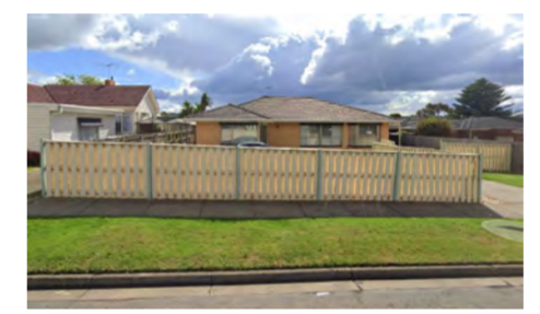
PHOTO 5 No 275 TORQUAY ROAD SINGLE BRICK DWELLING WITH TILE ROOF
