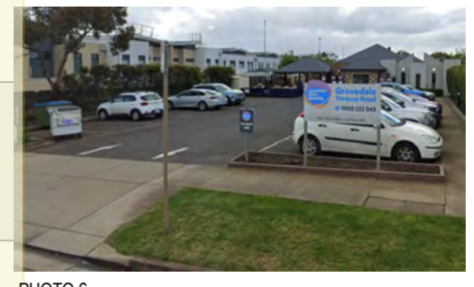
PHOTO 6 No 282 SINGLE STOREY BRICK AND RENDERED BUILDING C.I. ROOF EARLY START CHILD CARE CENTRE
