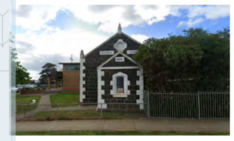
PHOTO 8 No 282 SINGLE STOREY BRICK AND RENDERED BUILDING C.I. ROOF EARLY START CHILD CARE CENTRE
