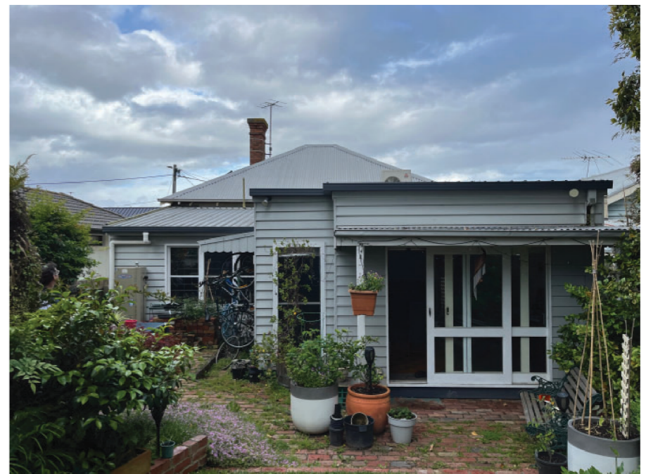
6. View of existing rear extension to be demolished.
