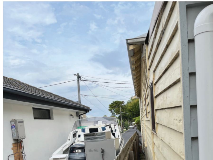
5. View along north boundary from rear towards Summer St.
