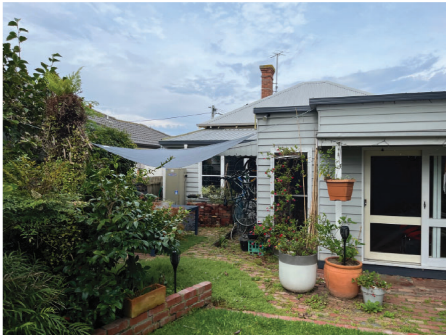
1. View of existing rear extension..
