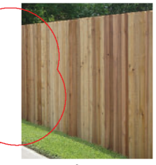
F - Boundary Fence Timber
