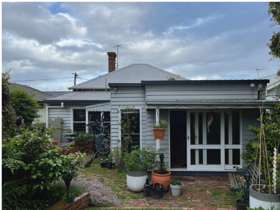
4. View of existing rear extension.
