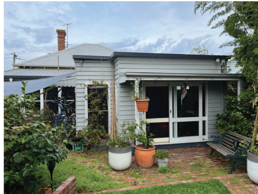
2. View of existing rear extension.
