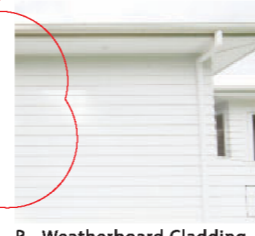
B - Weatherboard Cladding
