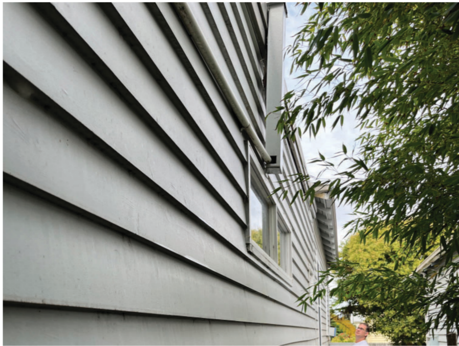
1. View of existing dwelling along south boundary.
