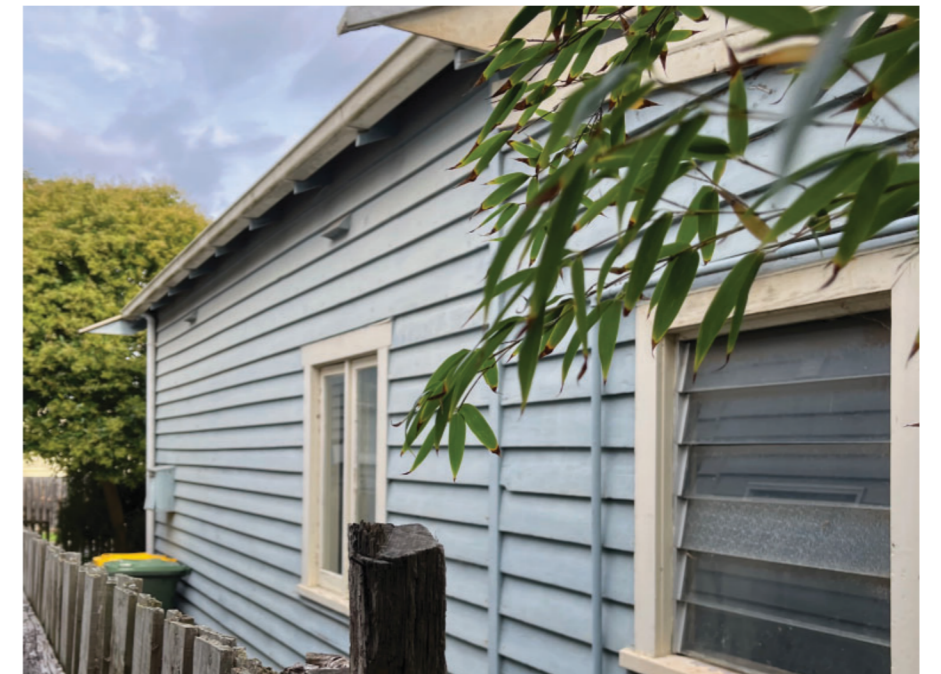
6. View of adjoining property to south.
