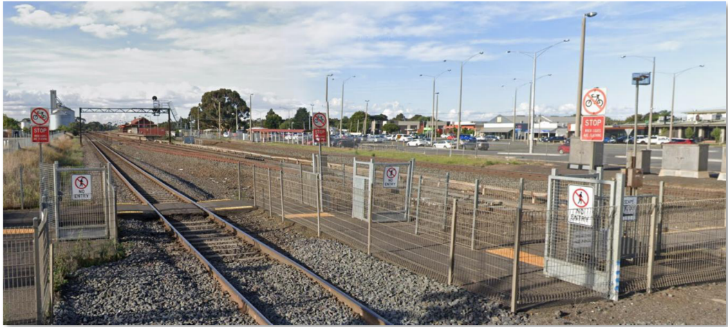
Image 6 - Railway land located to east of site
