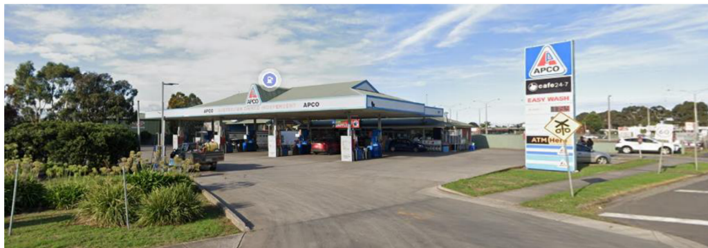
Image 14 - Existing signage viewed from Mill Road/ McClelland Avenue intersection
